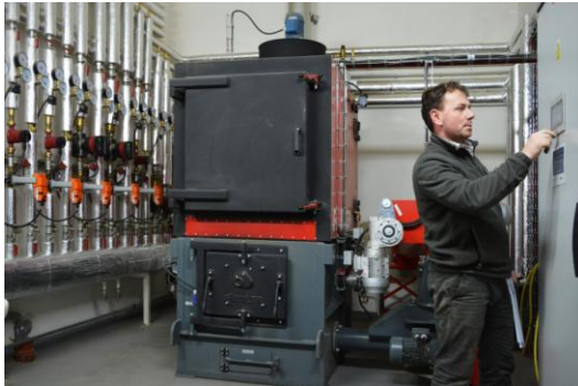
Automatic boiler room for wood biomass 2014
